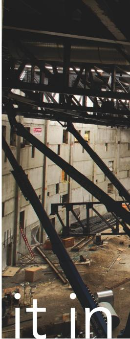
YOU KNOW IT'S A GREAT DAY when you top out a 4,600-ton structural steel project by dropping a 260-ft-long, 100-ton truss into place with 6 in. of clearance on either end, the client and other project big-wigs are watching, and the whole operation not only goes off without a hitch, but almost looks easy.
