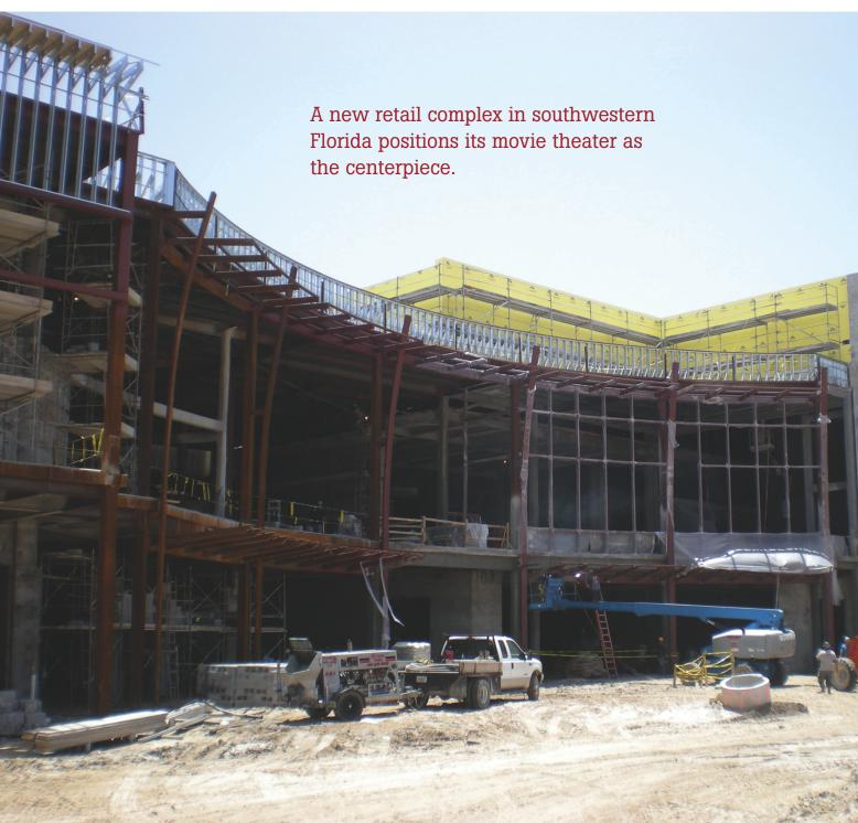
Entrance framing for Mercato's Building 8. Bracing locations were carefully coordinated with the theater above and retail below, placing most lateral resistance inboard of the façade to facilitate retail storefront exposure.
